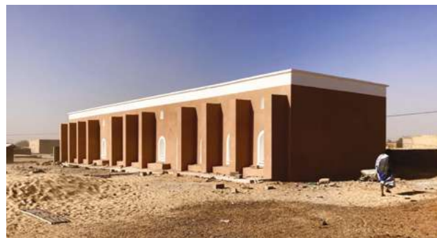
Fassala NV High School (▲ outside and ▼ inside).
