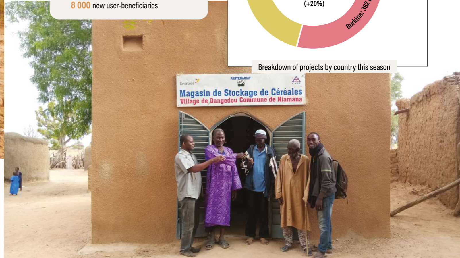
Delivery of the keys to the cereal storage building in Dangedou, Mali (SOS-Faim/CAEB project).
