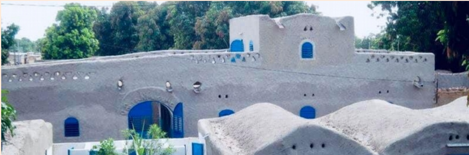
NV buildings in Boromo, Burkina Faso
