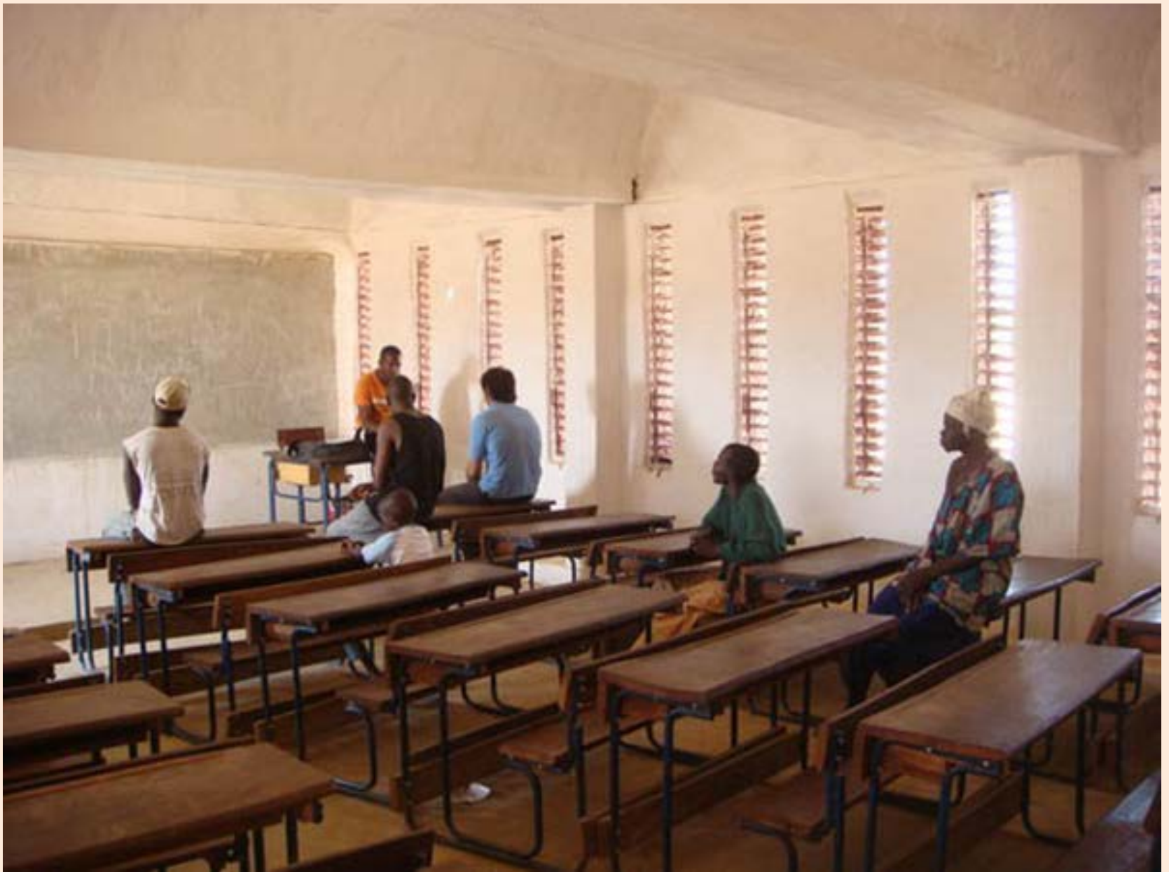
3 vault classroom, concrete post & beam, Djindjinebougou, Mali
