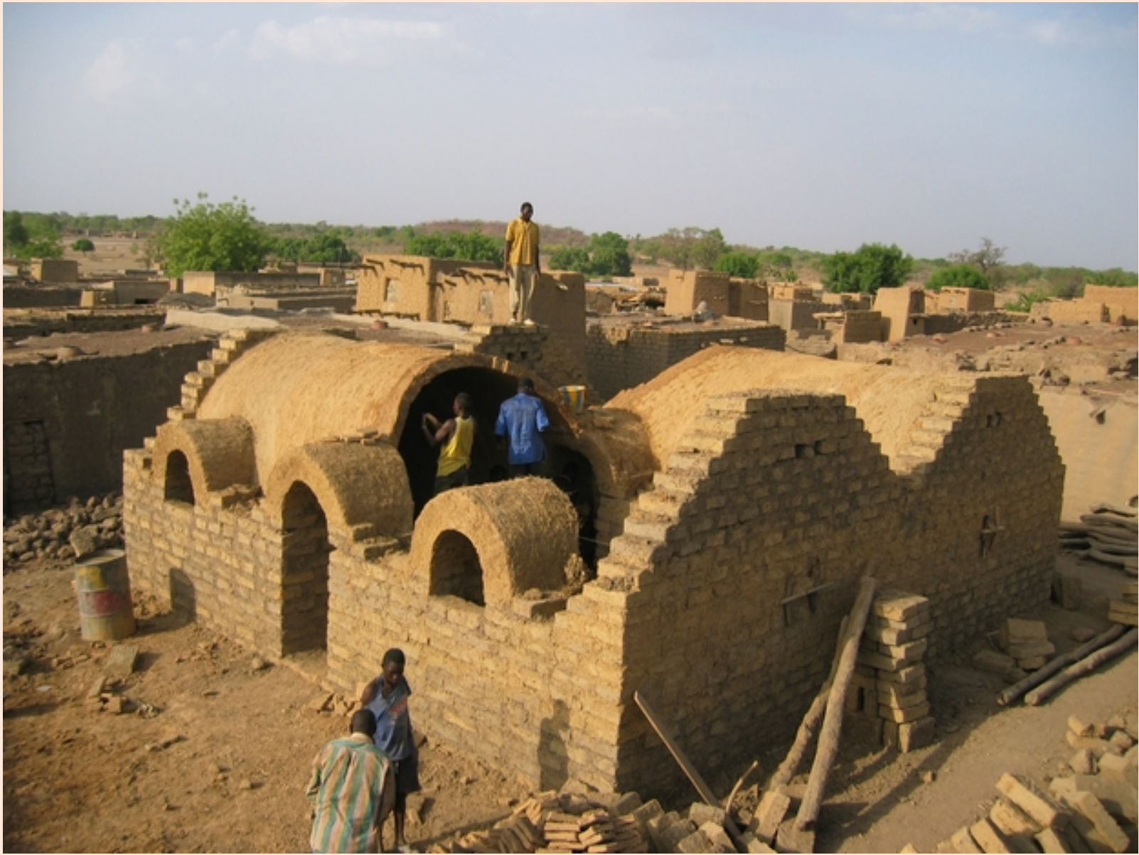
Twin-vault village house under construction, Burkina Faso
