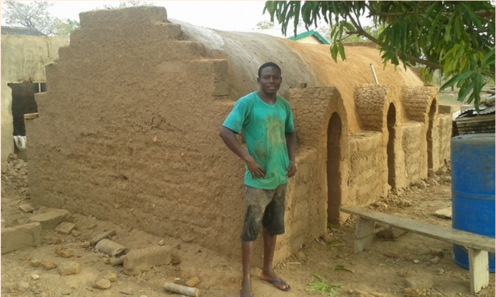
NV poultry shed, Ghana - 9% of NV buildings are for agricultural use - storage of crops, livestock ....
