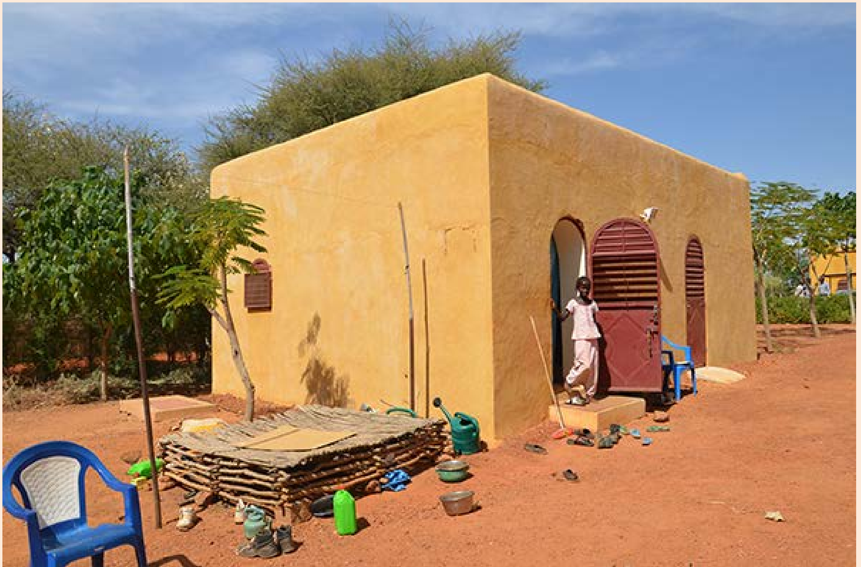
Single vault village house, Mali - 86% of NV buildings are houses for rural families, AVN's key target group
