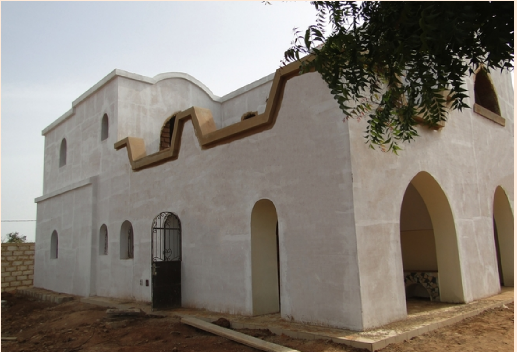
Cement render over 'stony' mud bricks, urban house, Senegal
