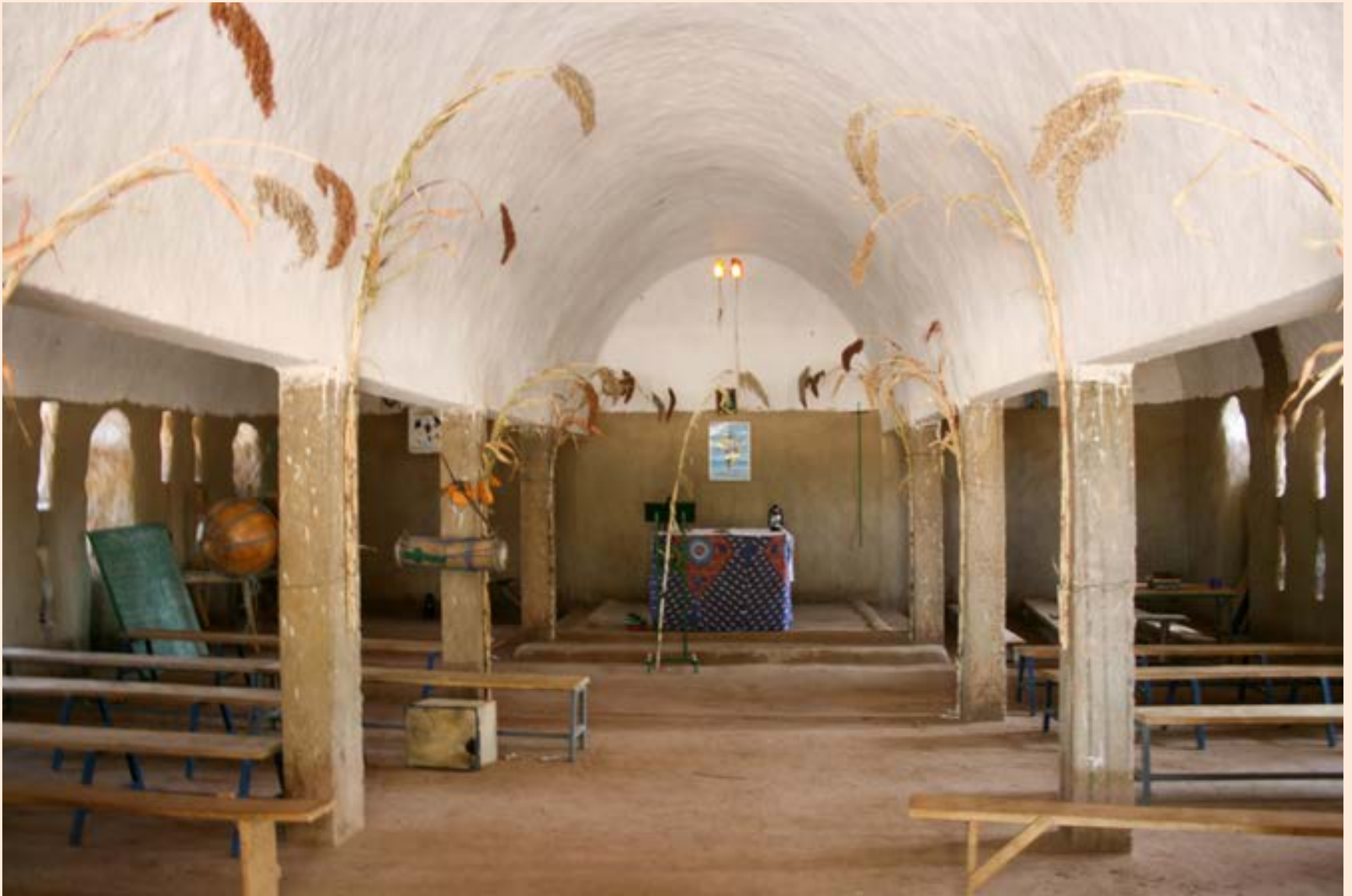
Reinforced concrete post & beam for church, Burkina Faso
