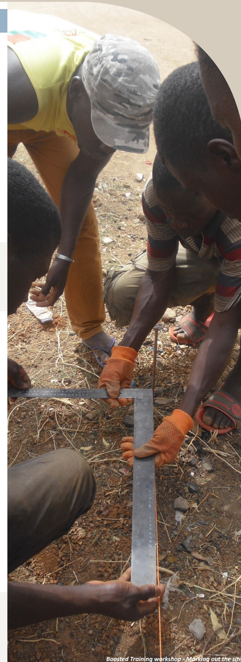
Boosted Training workshop - Marking out the site
