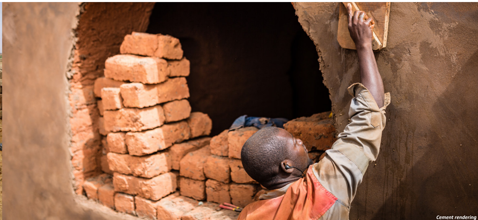
Construction of rammed earth foundations
