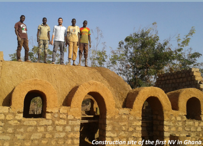
Construction site of the first NV in Ghana
